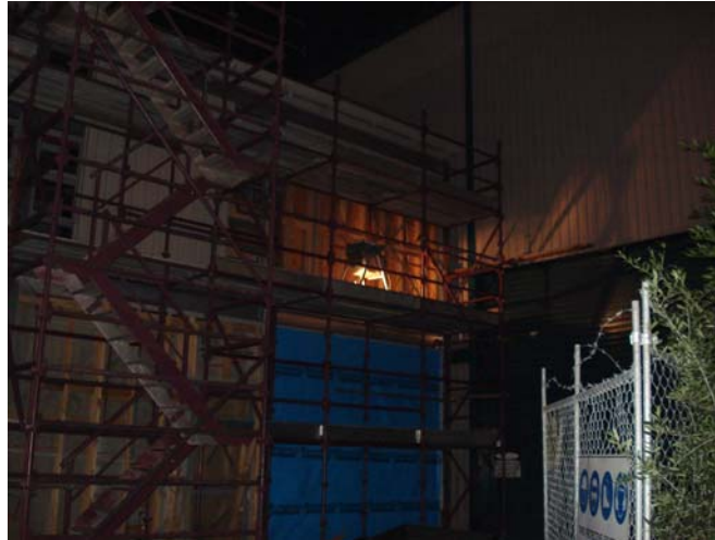
Figure 2. The outside of the STI screened room during attenuation testing. Accessed via the builder's scaffolding, the light shows the measurement equipment outside the screened room.
